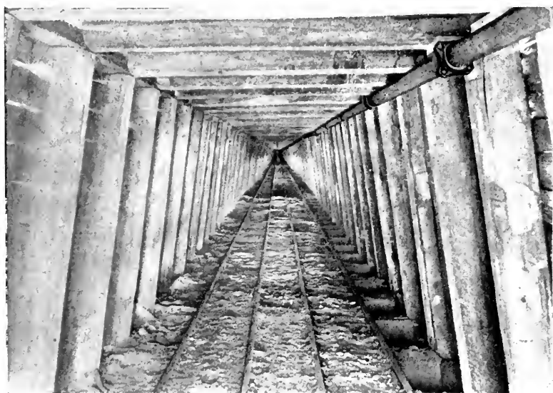
INTERIOR OF COWENHOVEN TUNNEL, OUTER 2000 FEET.
